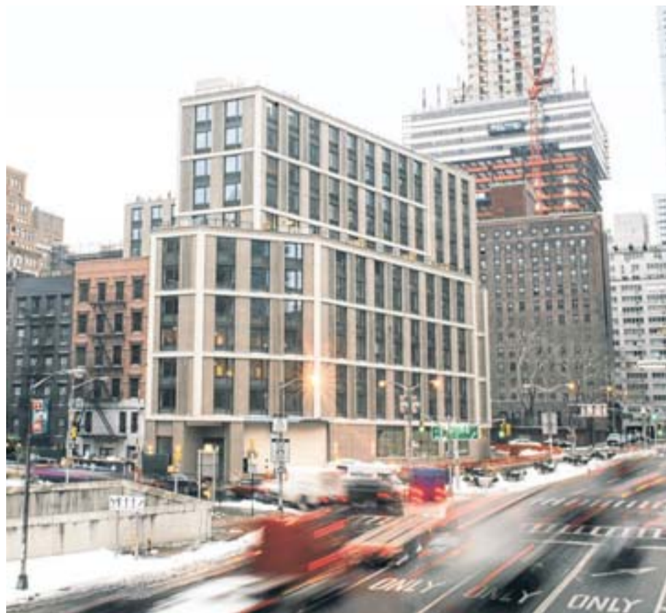
Developers of the Lewis, on West 35th Street, see the open space created by traffic lanes as an asset.
